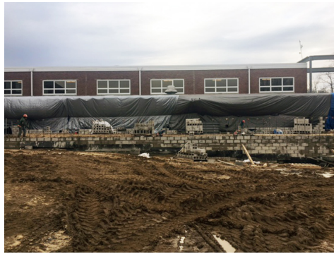
Above: Demolition of first floor science labs and construction of new outer walls in February 2018.
