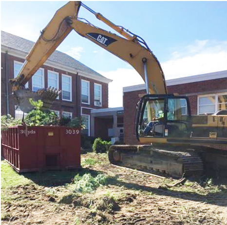
Above: Preparing the grounds by removing trees and shrubs back in October 2017.
