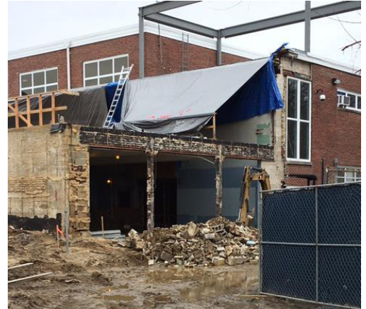
Above: Demolition of Room 202 and interior stairwell in February 2018.
